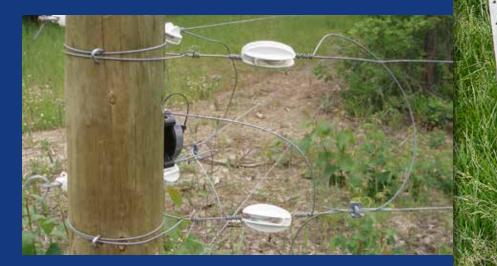
**Connect wires in parallel at the end of runs.** A good way to increase the ability of a fence to carry voltage is to connect all the wires at the beginning and end of runs of multi-wire fence. This allows the multiple strands of high tensile wire to function as one large wire that is capable of carrying higher levels of voltage.
