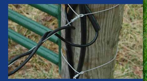
Always use underground cable designed for electric fencing and place it in protective tubing. It is very important to only use underground cable that is designed for electric fence. Never use any product that is intended for residential use. Whenever a cable carrying current is run under the ground, always place it in some type pipe or conduit that will protect it from future damage. Wires going under gates should be buried to a depth of approximately 1 foot.
