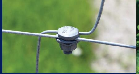
Always connect electrified wires with clamps. Loose connections result in loss of voltage. Connections should NOT be wrapped, but rather clamped together with a high-quality clamp that is designed for high tensile fencing. Never use clamps that are constructed of dissimilar metals. Although economy clamps constructed of cast metal are sometimes available, they often fail upon tightening. Saving a few cents on clamps often leads to exponential headaches in the future.
