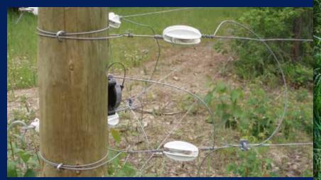
Connect wires in parallel at the end of runs. A good way to increase the ability of a fence to carry voltage is to connect all the wires at the beginning and end of runs of multi-wire fence. This allows the multiple strands of high tensile wire to function as one large wire that is capable of carrying higher levels of voltage.
