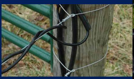
Always use underground cable designed for electric fencing and place it in protective tubing. It is very important to only use underground cable that is designed for electric fence. Never use any product that is intended for residential use. Whenever a cable carrying current is run under the ground, always place it in some type pipe or conduit that will protect it from future damage. Wires going under gates should be buried to a depth of approximately 1 foot.
